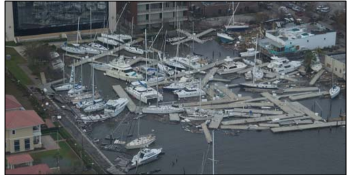
2004: Heavy damage from Hurricane Ivan to a Florida marina. Photo by PA3 Andrew Kendrick.
